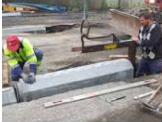
Installation team – two men plus lifting tool lay the pipes in a work trench 80 cm wide
