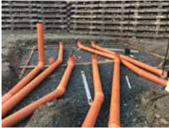
Connecting pipes to fans and siphon pot
