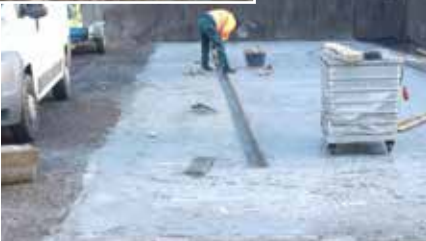
Reconditioned decomposition area with in-floor concrete aeration pipes
