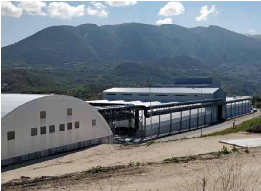
Box composting – drying box with integrated energy recovery from CHP waste heat (biogas plant) in Epirus, Greece
