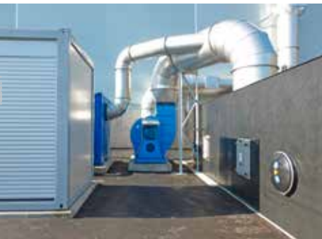
Hrastnik composting plant Construction period: approx. 12 months Operation since: Winter 2015/2016 Input: 6,000 t/year MSW, 6,000 t/year biowaste Technical equipment: 6 negative-aerated MSW windrows 4 negative-aerated biowaste windrows, positive-aerated curing phase for biowaste Turner: TracTurn Scope of delivery: engineering, aeration technology, EI&C, exhaust air system, TracTurn
