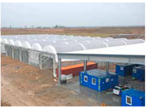
Construction period: approx. 8 months Operation since: Spring 2016 Input: 60,000 t/year MSW Technical equipment: 11 positive-aerated composting tunnels, non-aerated curing phase Turner: CMC SF 300 Scope of delivery: engineering, aeration technology EI&C, box systems, CMC SF 300
