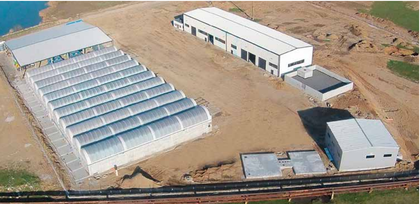
Construction period: approx. 8 months Operation since: Spring 2016 Input: 60,000 t/year MSW Technical equipment: 11 positive-aerated composting tunnels, non-aerated curing phase Turner: CMC SF 300 Scope of delivery: engineering, aeration technology EI&C, box systems, CMC SF 300
