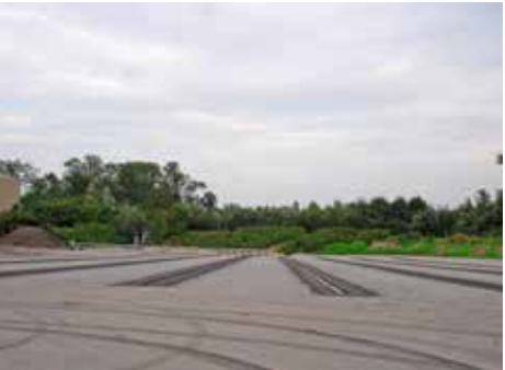
The "COMPOnent" aeration system was installed on the first composting plant in Austria in 1997. Today an annual volume of over 160,000 tons of sewage sludge is composted throughout Austria on 15 composting plants.
