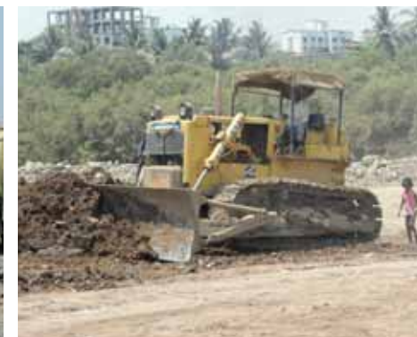
With daily more than 1,000 tons of excavated earth the construction land was risen approximately 4 m. In the background „THE WALL“! At a length of more than 5 km, the wall surrounding the Kanjur facility is a record in itself. Using the simplest of means, even the concrete blocks were manufactured in the facility.
