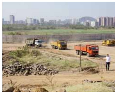
With daily more than 1,000 tons of excavated earth the construction land was risen approximately 4 m. In the background „THE WALL“! At a length of more than 5 km, the wall surrounding the Kanjur facility is a record in itself. Using the simplest of means, even the concrete blocks were manufactured in the facility.
