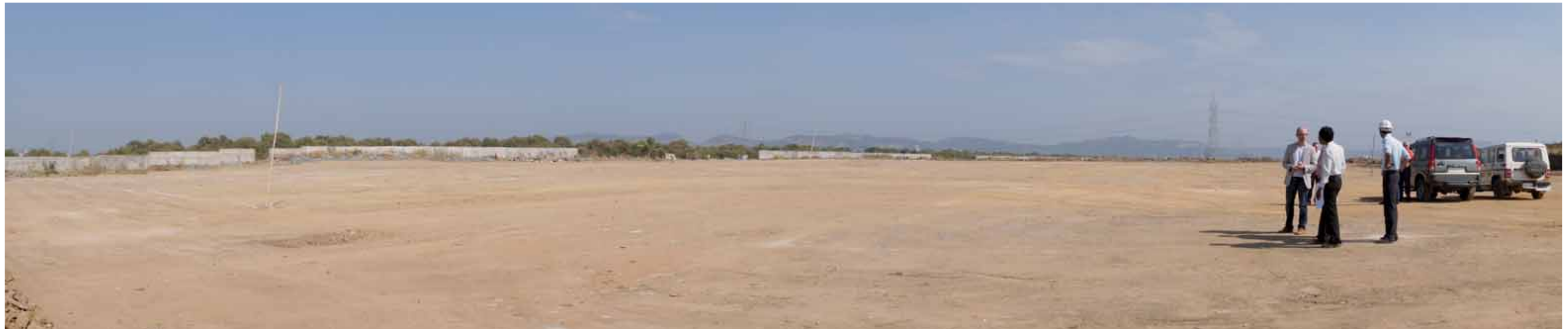
With daily more than 1,000 tons of excavated earth the construction land was risen approximately 4 m. In the background „THE WALL“! At a length of more than 5 km, the wall surrounding the Kanjur facility is a record in itself. Using the simplest of means, even the concrete blocks were manufactured in the facility.
