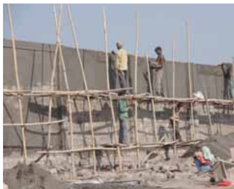
With daily more than 1,000 tons of excavated earth the construction land was risen approximately 4 m. In the background „THE WALL“! At a length of more than 5 km, the wall surrounding the Kanjur facility is a record in itself. Using the simplest of means, even the concrete blocks were manufactured in the facility.
