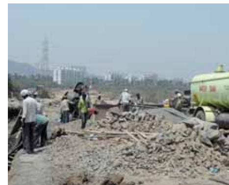
With daily more than 1,000 tons of excavated earth the construction land was risen approximately 4 m. In the background „THE WALL“! At a length of more than 5 km, the wall surrounding the Kanjur facility is a record in itself. Using the simplest of means, even the concrete blocks were manufactured in the facility.
