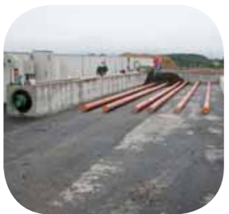
...building the biofilter
