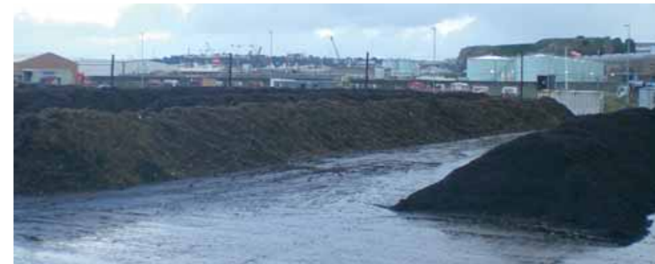
20 temperature probes help in odour reduction at the compost plant "Jersey" on the Channel Islands – Turning takes place dependent on the windrow temperature
