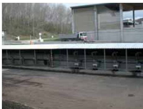
Blower station MBT plant
