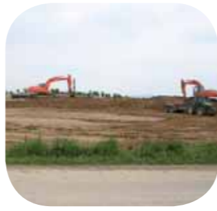
30.000 m 3 of earthworks to be managed
