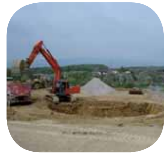
leachate storage and push wall
