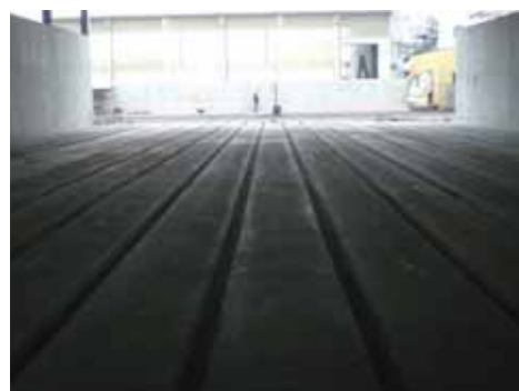
Finished composting area MBT
