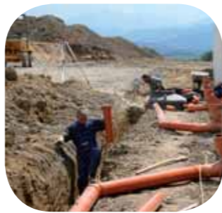
hauling of the pipes...
