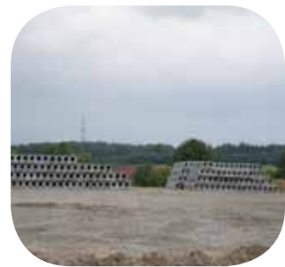
finally - COMPOair, the heart of the aeration equipment, was delivered
