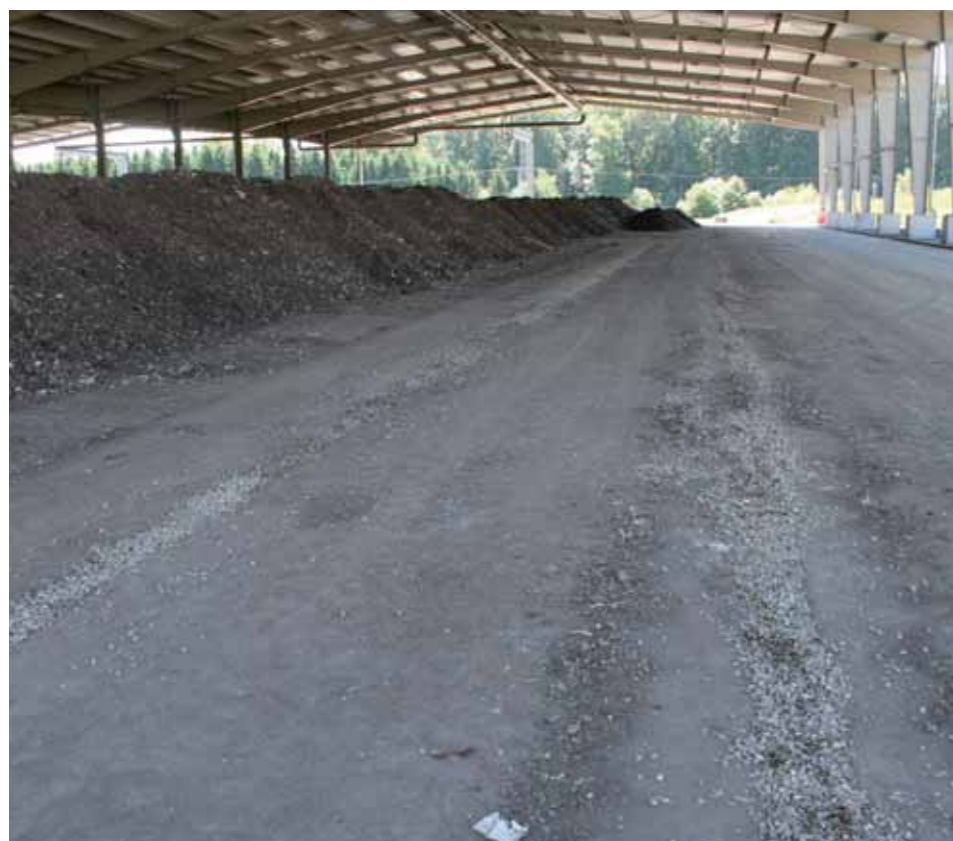
Looking into the compost hall
