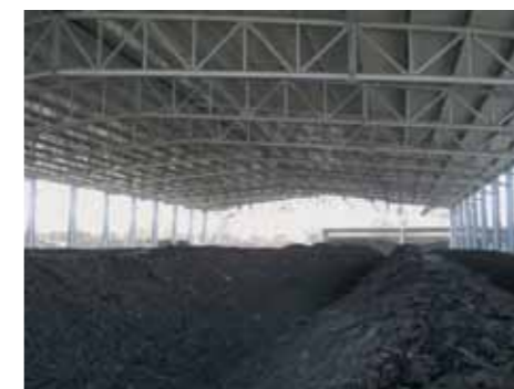
Looking into the compost hall
