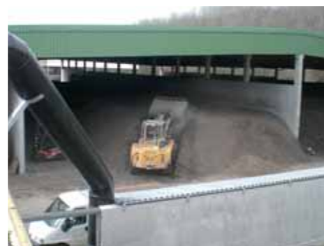
Building of the MBT windrow
