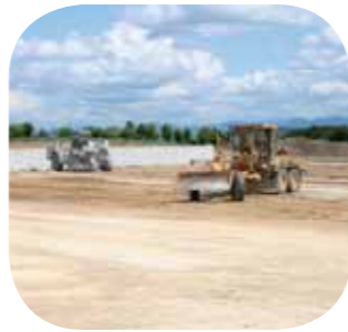
unexpected difficulties - the floor needs to be stabilized with lime
