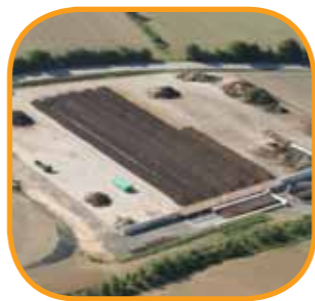
...and finally after only three months building - DONE!
