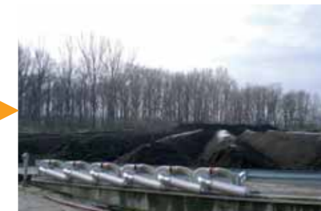
Finished compost plant
