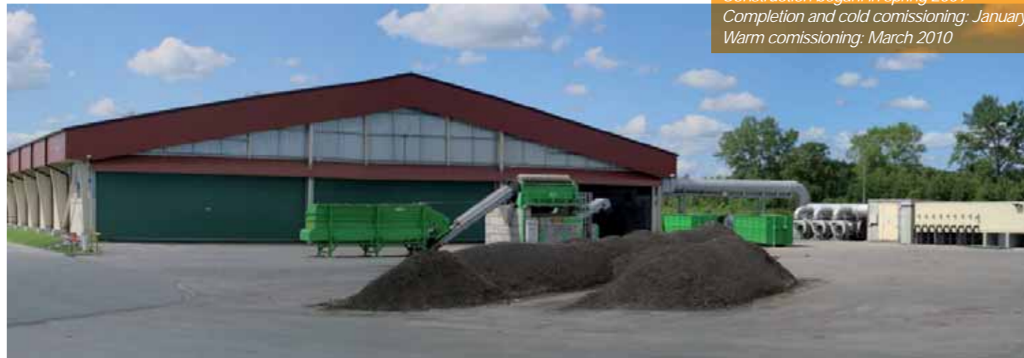
Compost hall with screening station, curing area and biofilter
