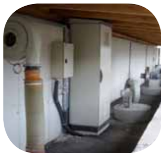
... connecting fans and controlling system...
