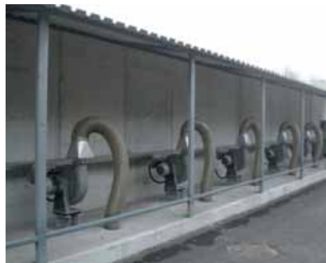
Blower station green waste compost
