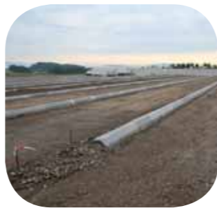
...the eight aeration rows are laid and the area can be paved
