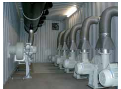
Pre-mounted fan container
