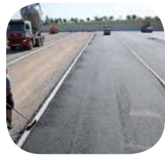
base course and sealing tarmac...
