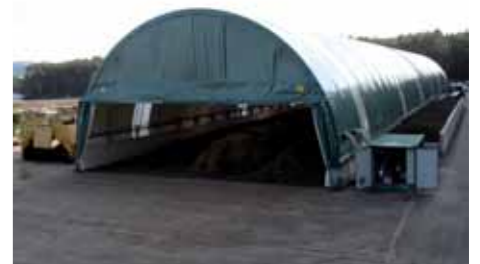
Compact construction method
