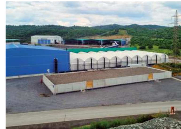
Anlage in Tripoli.
