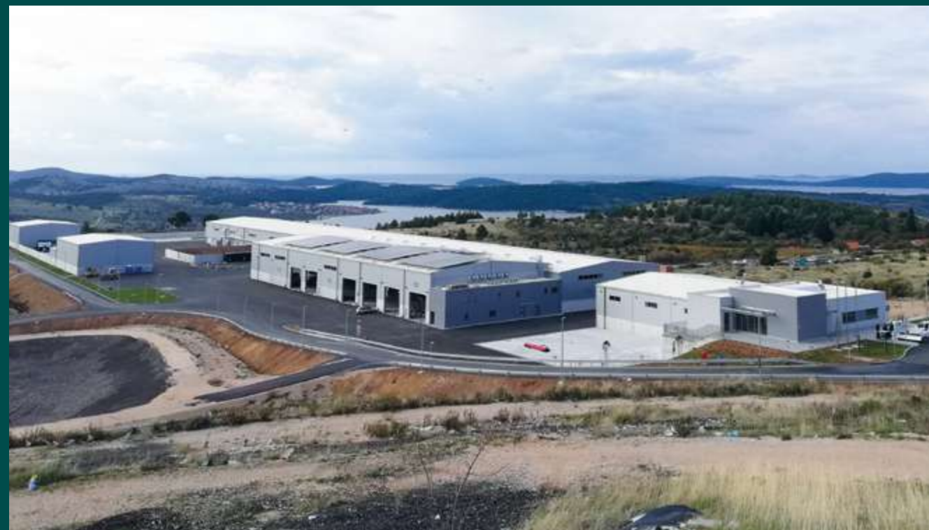
The CGO Bikarac composting plant has already been in full operation since 2022 and processes 43,000 tonnes of biowaste and household waste per year.
