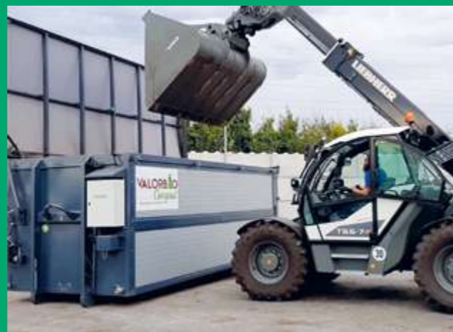
Filling the CSC-Container using a telescopic handler.
