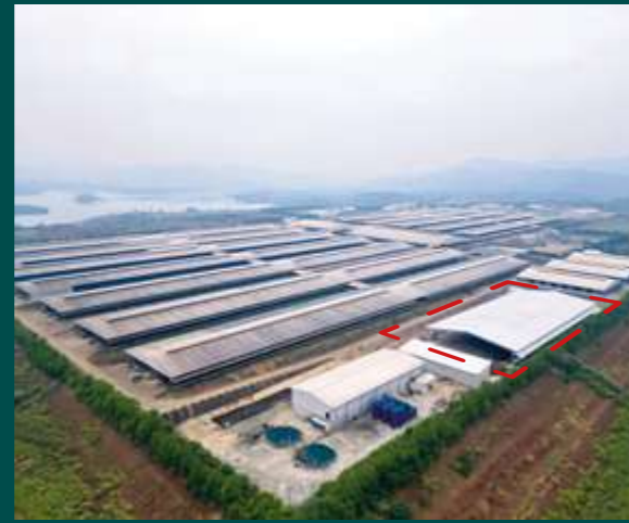
Barns (in the background) and composting plant in Thanh Hóa. The composting hall (marked in red) measures 40 x 100 m.
