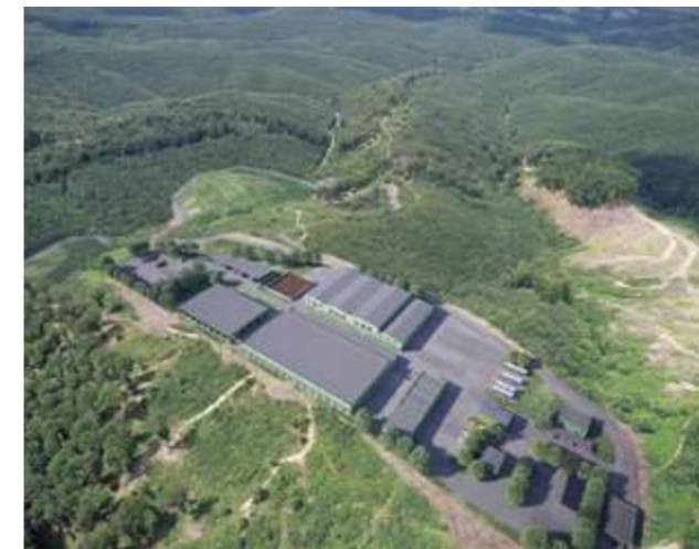
Aerial view of the Babina Gora composting plant.
