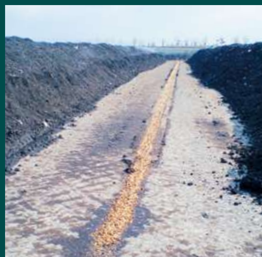
An aeration line at the composting plant.
