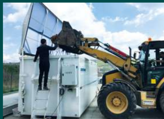
Filling the CSC-Container using a wheel loader.
