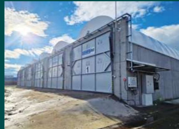
Waste is composted in enclosed boxes.
