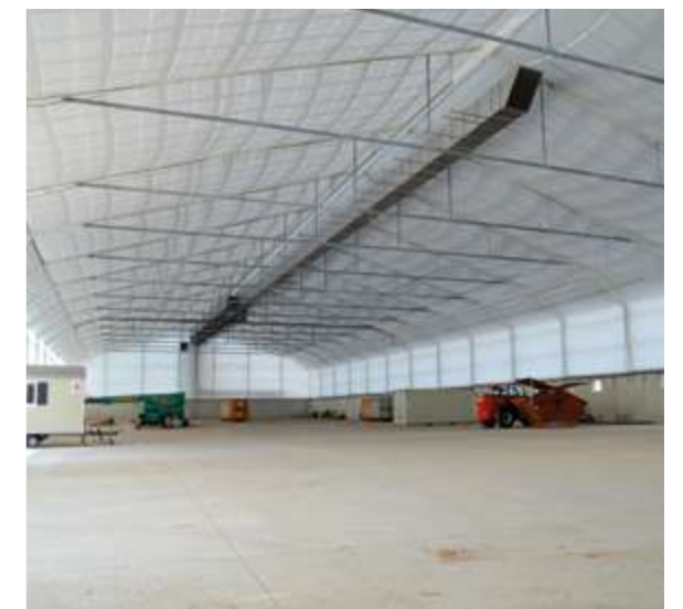
Thanks to the light-transmitting roof design, no lighting is required during the day.
