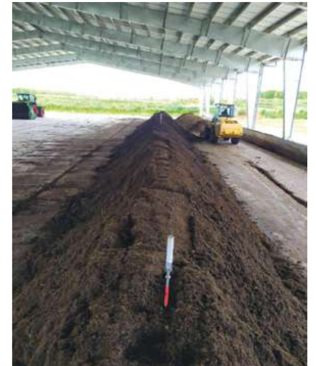
Building and automated temperature monitoring of the first windrows at the plant in Phú Yên.
