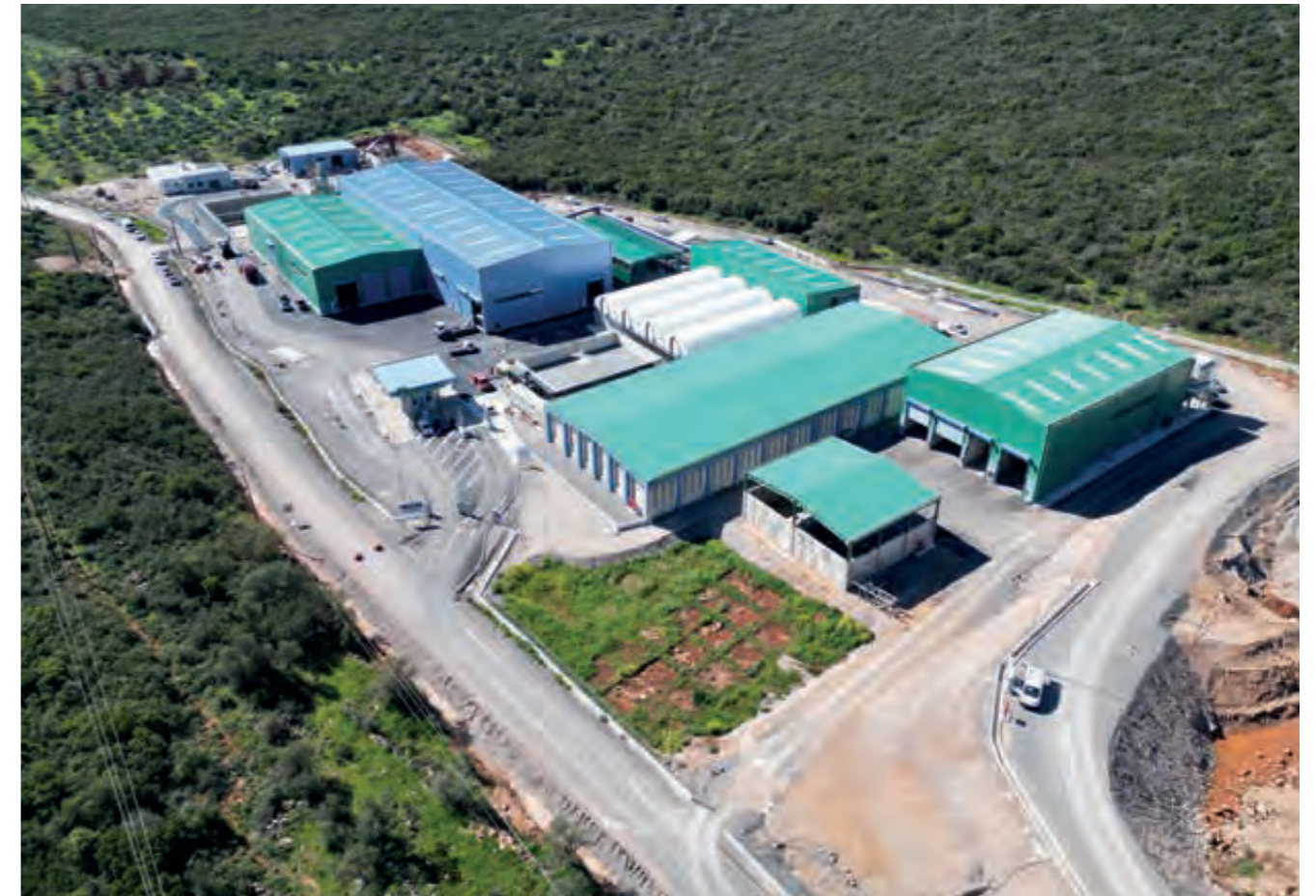
The plant in Sparta is already in full operation.
